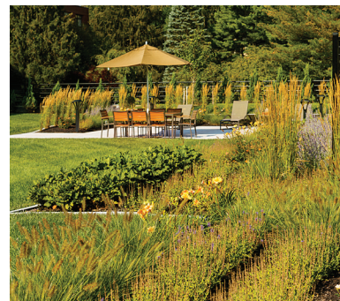
Top left to bottom right: Recover led soil conveyors to move over 1,000 yards of media onto the roof, and graded it to depths of three feet / Recover installed over 8,000 square feet of color-ground pavers and granite curbing / Two dozen species of perennials were planted to create a lush English-style garden // Images by Patrick Rogers Photography
